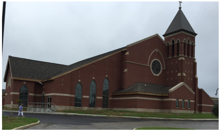
Exterior: St. Mary, Greensburg
